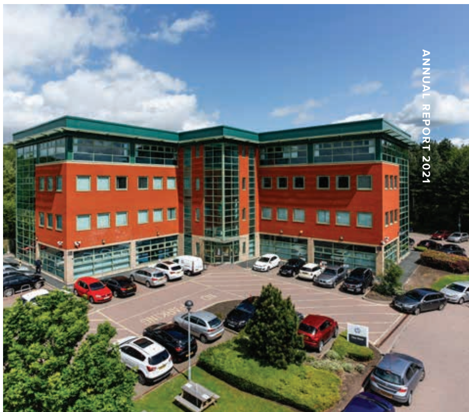
TITAN HOUSE, TELFORD
