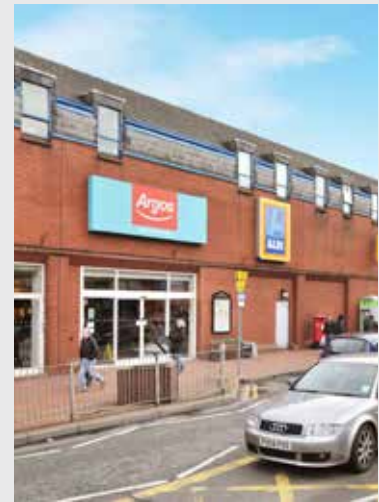
BEARWOOD ROAD SHOPPING CENTRE
